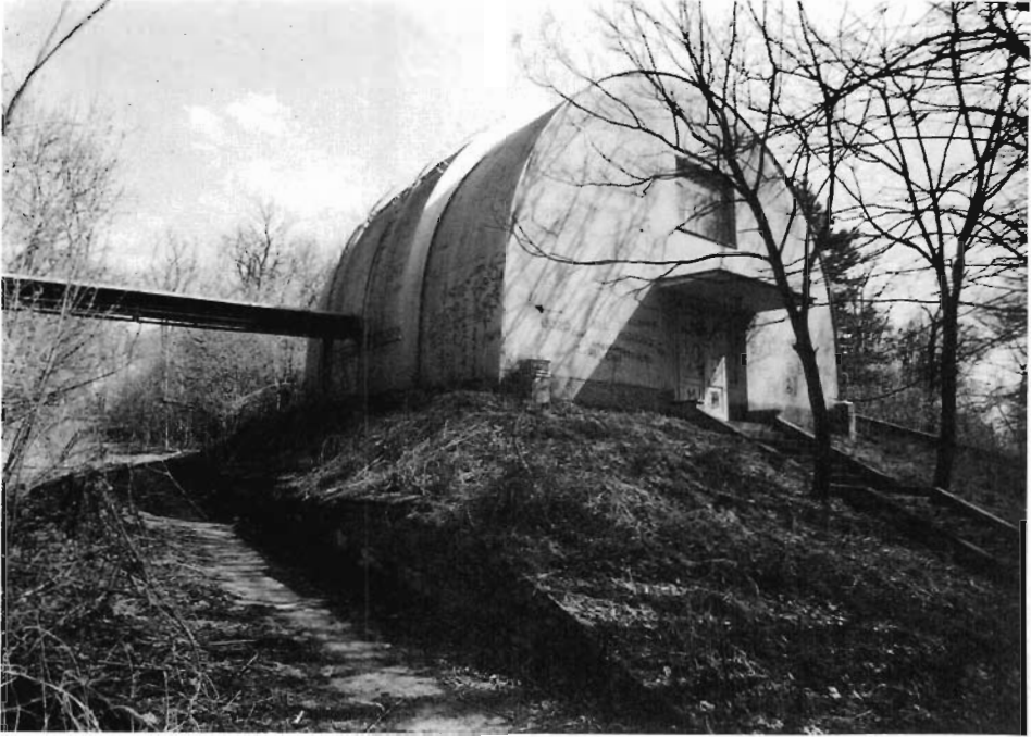
Fig. 17. The pavilion of the Large Transit Instrument. Visible parts of vacuum tubes connective meridian marks with the instrument.
